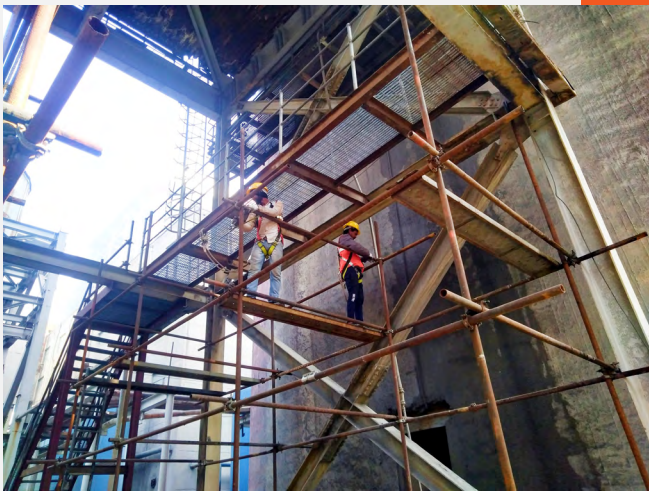
Use of tool tie at higher elevations to prevent tools from falling
