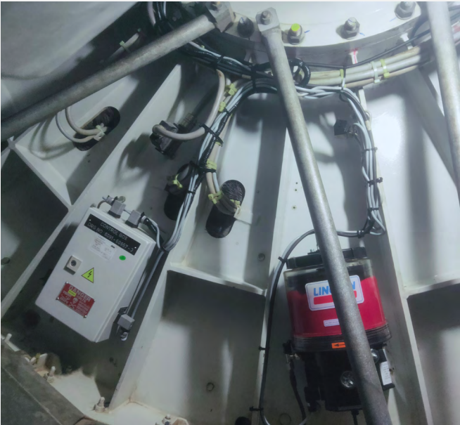
Installed CLS system in Spinner Area of WTG
