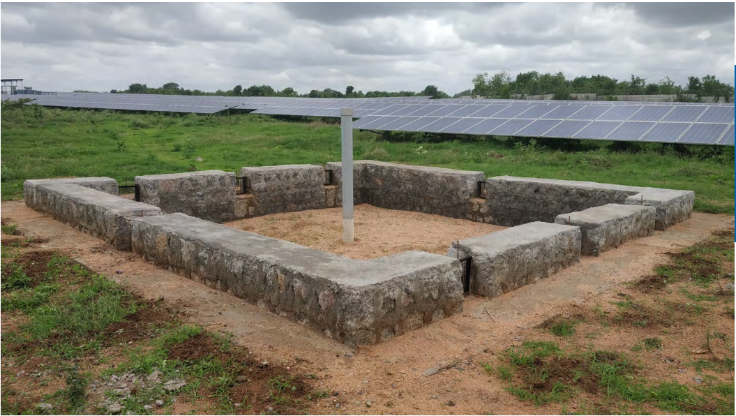
Rainwater Harvesting Structure at DSPL solar site
