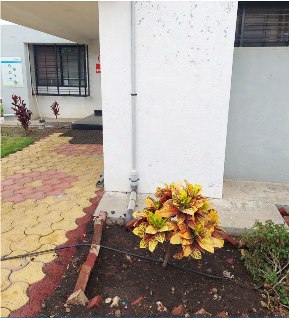
Rooftop Rainwater Harvesting at Khandke wind site
