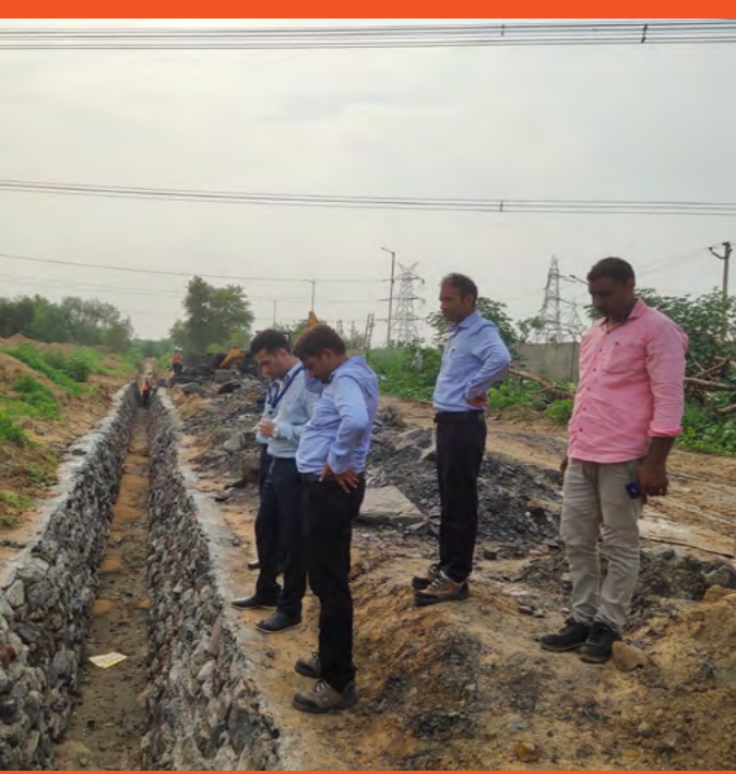
In-house Wetland Drain Under Construction
